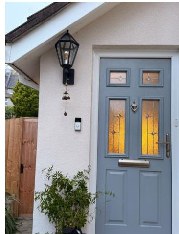
3. Completed Isolocork finish.
