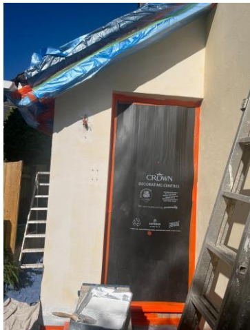
1. Existing lime-rendered wall prepared and repaired.
