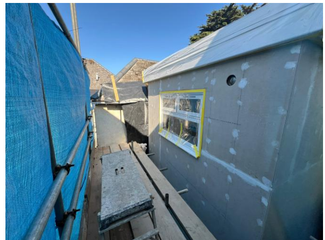
2. CMC carrier board installed and joints/fixings prepared.
