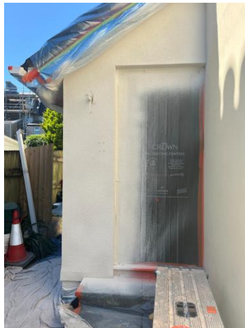
2. Isolocork application following preparation and primer.
