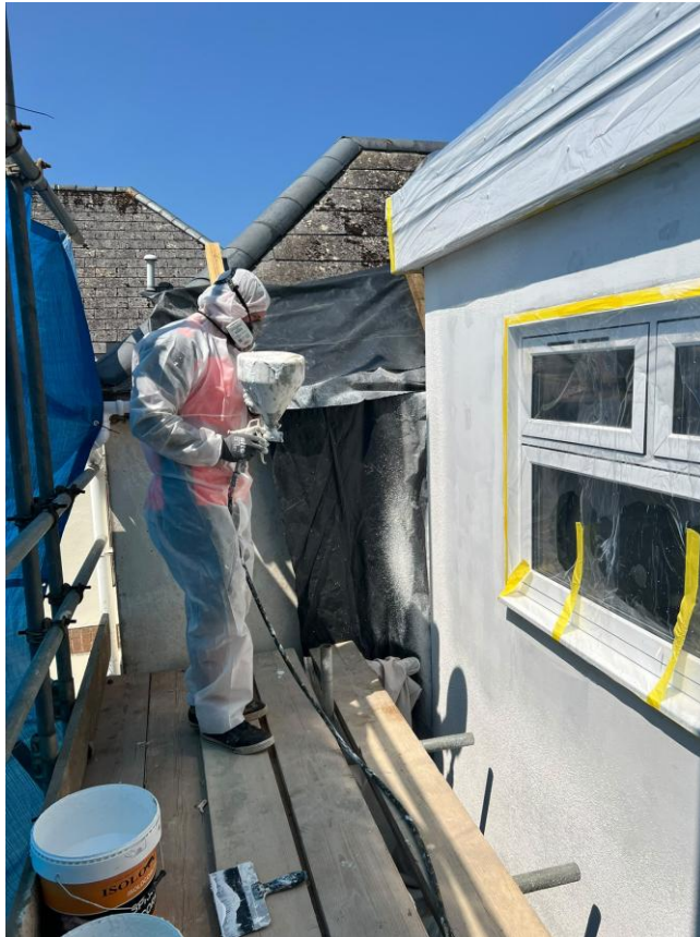
3. Isolocork Spray Cork being spray-applied.
