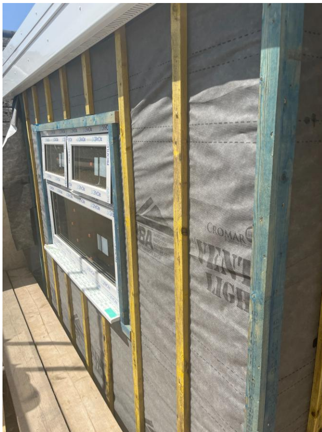
1. Timber structure, breather membrane and battens.
