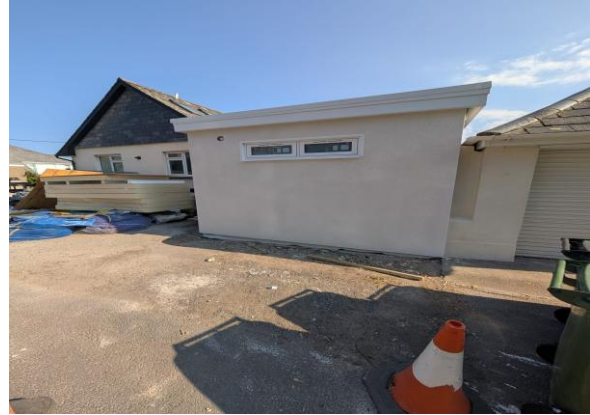
Completed extension Completed Woolacombe extension with the Isolocork external finish.
