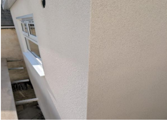
Finished surface Close view showing the continuous textured Isolocork finish.
