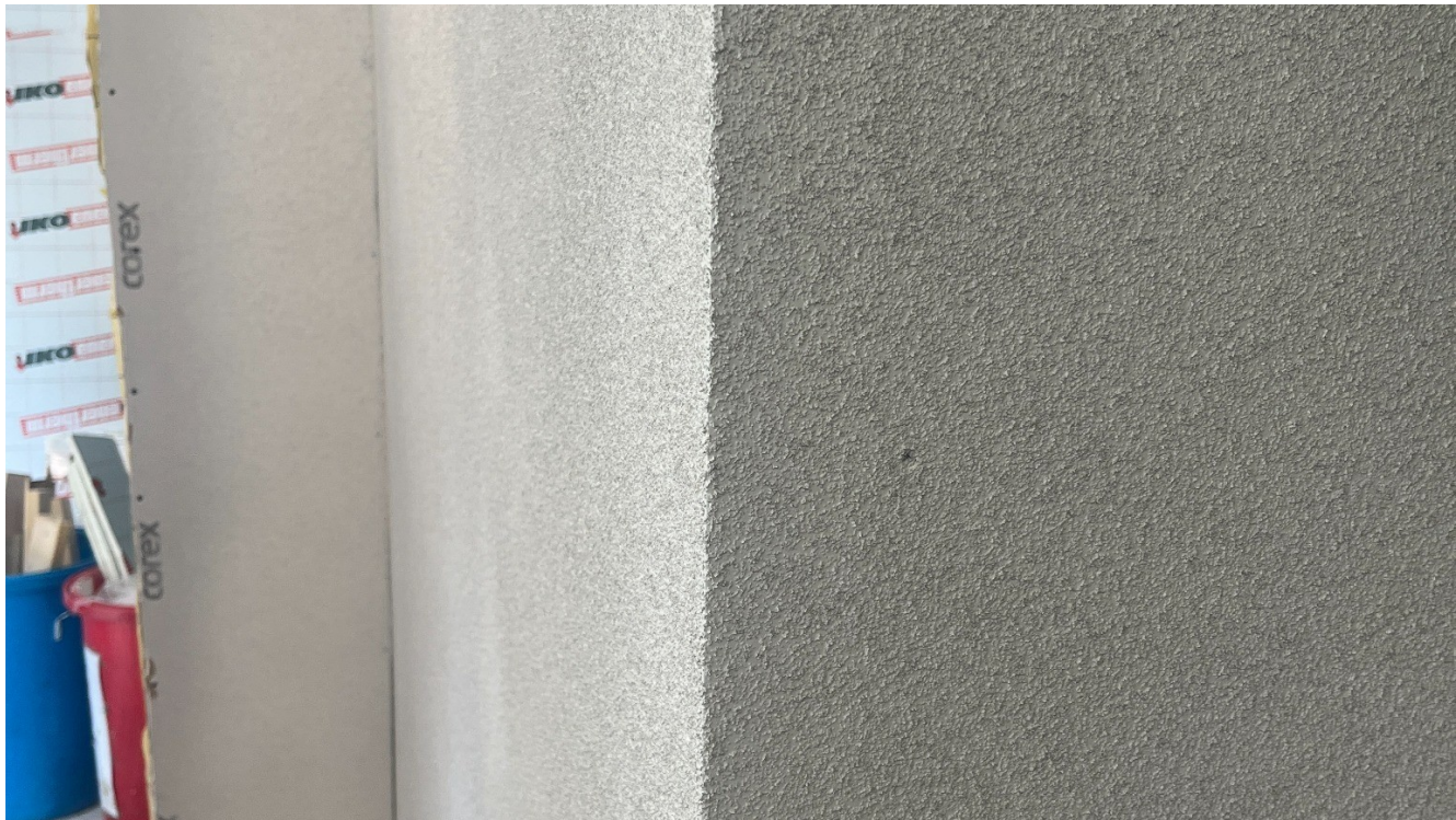
Internal Isolocork application carried out in Livingston during a practical training session.
